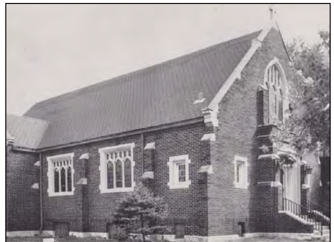
Bethel building—dedicated October 1930
